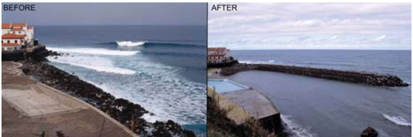
Coastal protection schemes can result in the loss of surf breaks, as seen here at Ponta Delgada, Madeira. Photo courtesy of Save The Waves ( www.savethewaves.org ).
