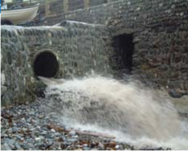
Combined storm overflows can discharge raw sewage directly onto beaches in heavy rain.
